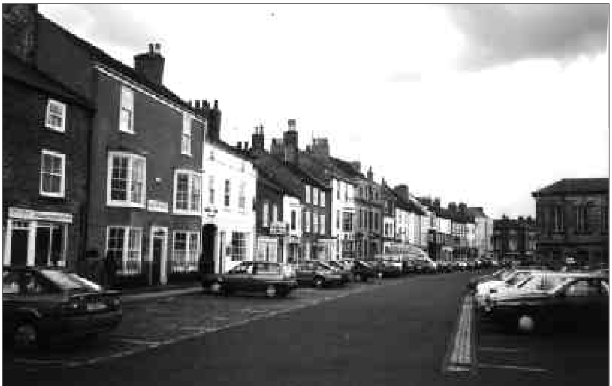
High Street looking west towards the Town Hall
